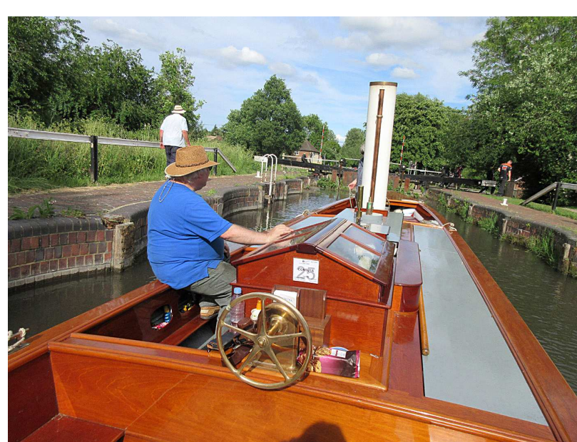
Above:- Aldermaston lock is about 110ft long and 18ft wide with a rise of 9ft, Originally a turf sided lock but was restored to full side height by BW in 1986 and is now a listed structure.
