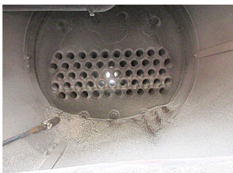
Top left:- High pressure jet wash
