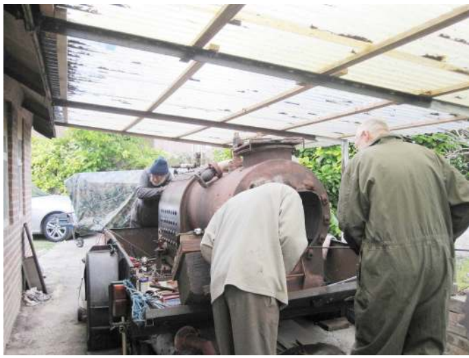
Needle gun cleaning below.
