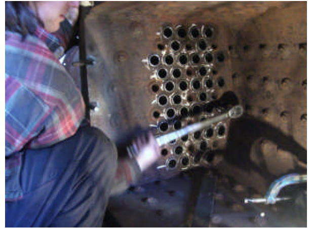
On the left the first part of the expanding operation can be done with an electric drill but the final expanding drive is manual using a torque lever because of the high torques needed and to get the right amount of tube expansion. The torque setting for these tubes was 50 ftlbs.
