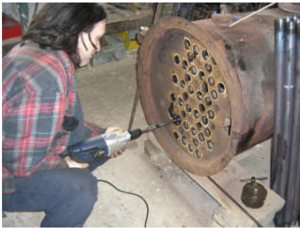
On the left the first part of the expanding operation can be done with an electric drill but the final expanding drive is manual using a torque lever because of the high torques needed and to get the right amount of tube expansion. The torque setting for these tubes was 50 ftlbs.
