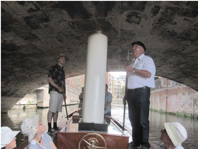
Reading High street bridge - checking clearance
