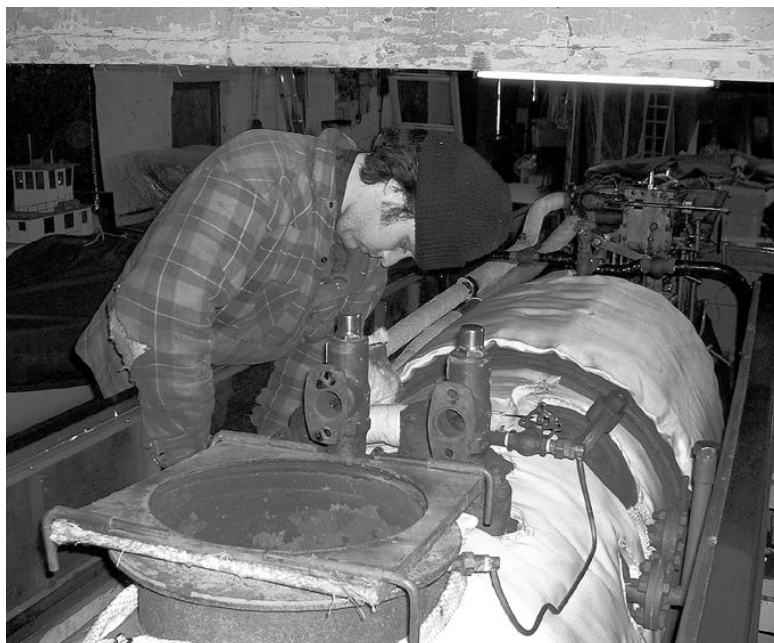
Fitting the boiler lagging
